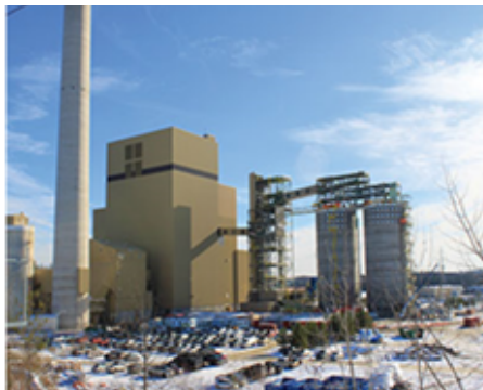
ATIKOKAN Closed 2013, converted to biomass and reopened 2014.
