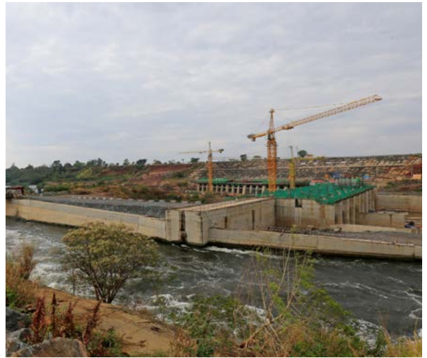
Karuma Hydro Dam, Uganda
