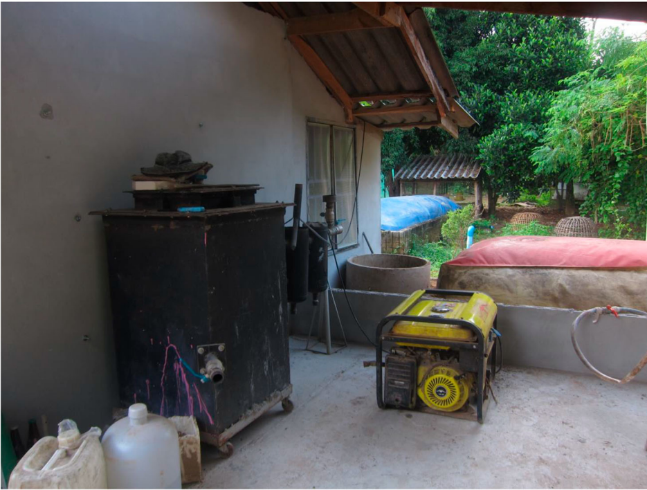
Figure 3. The biogas produced from the balloon-type biogas digester (shown in orange and blue coloured polyethylene plastic materials) can be connected to a generator set (the yellow equipment in the centre of the photograph) to generate electricity supplementing energy generated from a solar home system. Source: Photographed by the author, November 2016.
