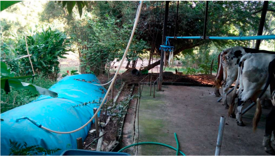
Figure 2. The Pa Deng biogas digester is an innovation from classic brick or concrete digesters. Source: Photographed by the author, November 2016.
