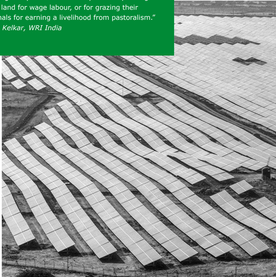
Solar panels Pavagada in Tumakuru district of Karnataka (photo credits: Pushkar V via Flickr.com)
