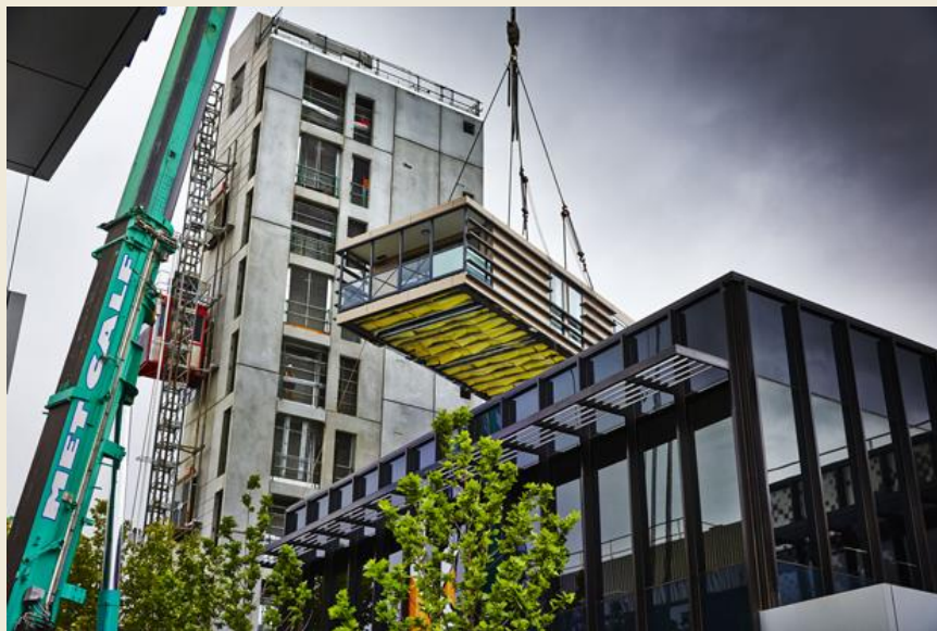
Little Hero on site construction
