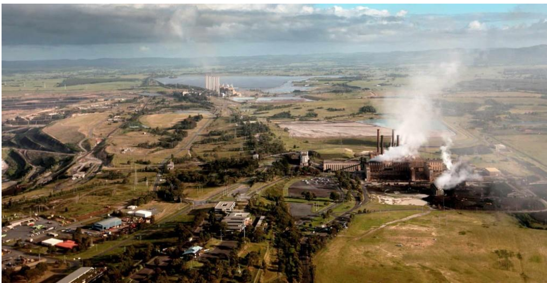
Aerial view of Hazelwood power station and retired Energy Brix factory
