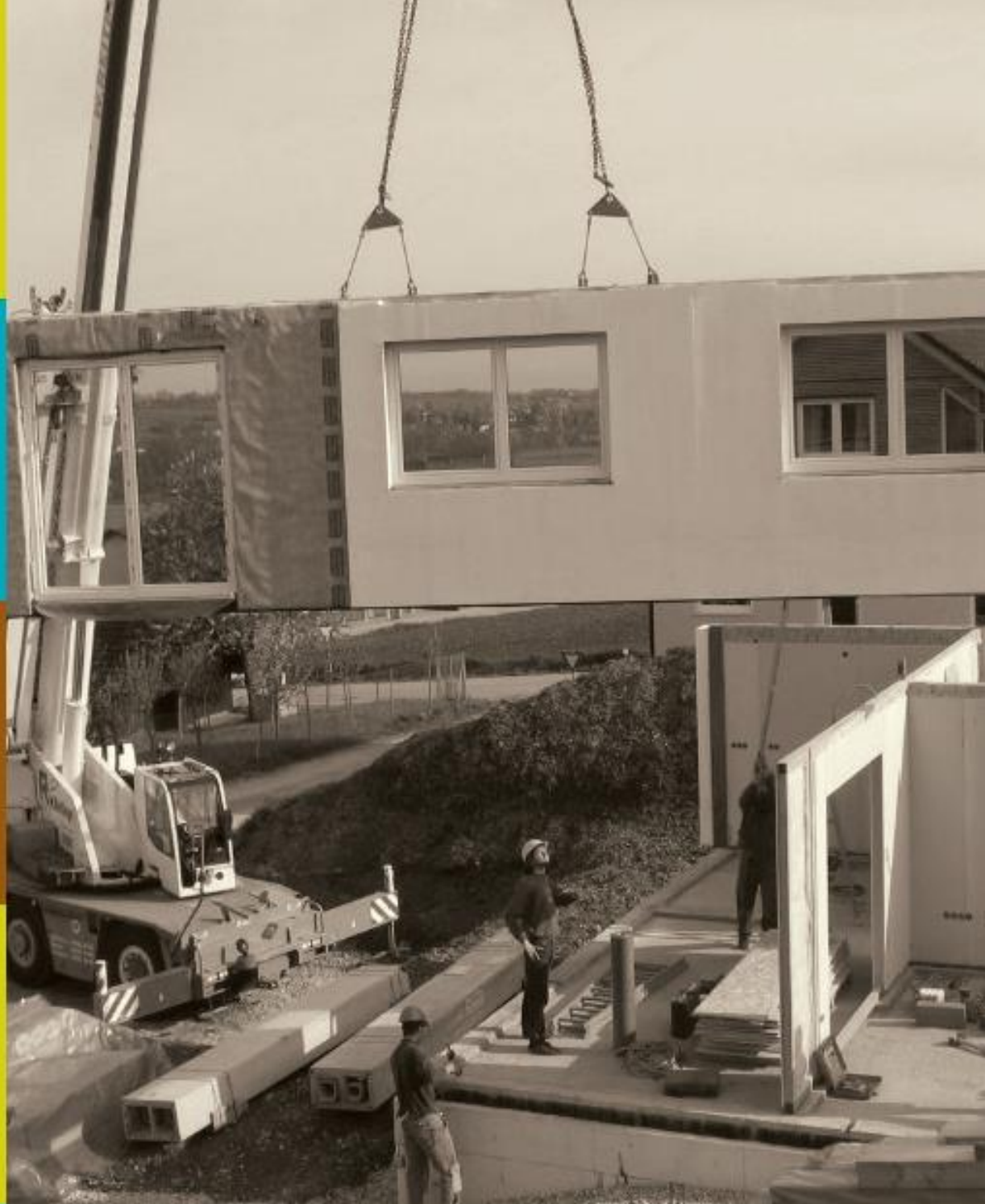
Above: Workers in the UK construct a prefabricated house
