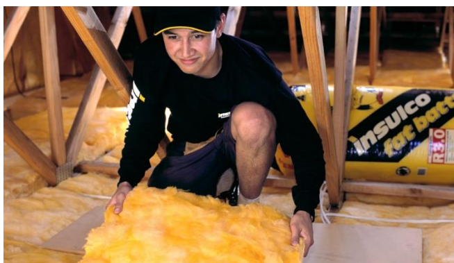
Insulco employee installs roofing insulation.
