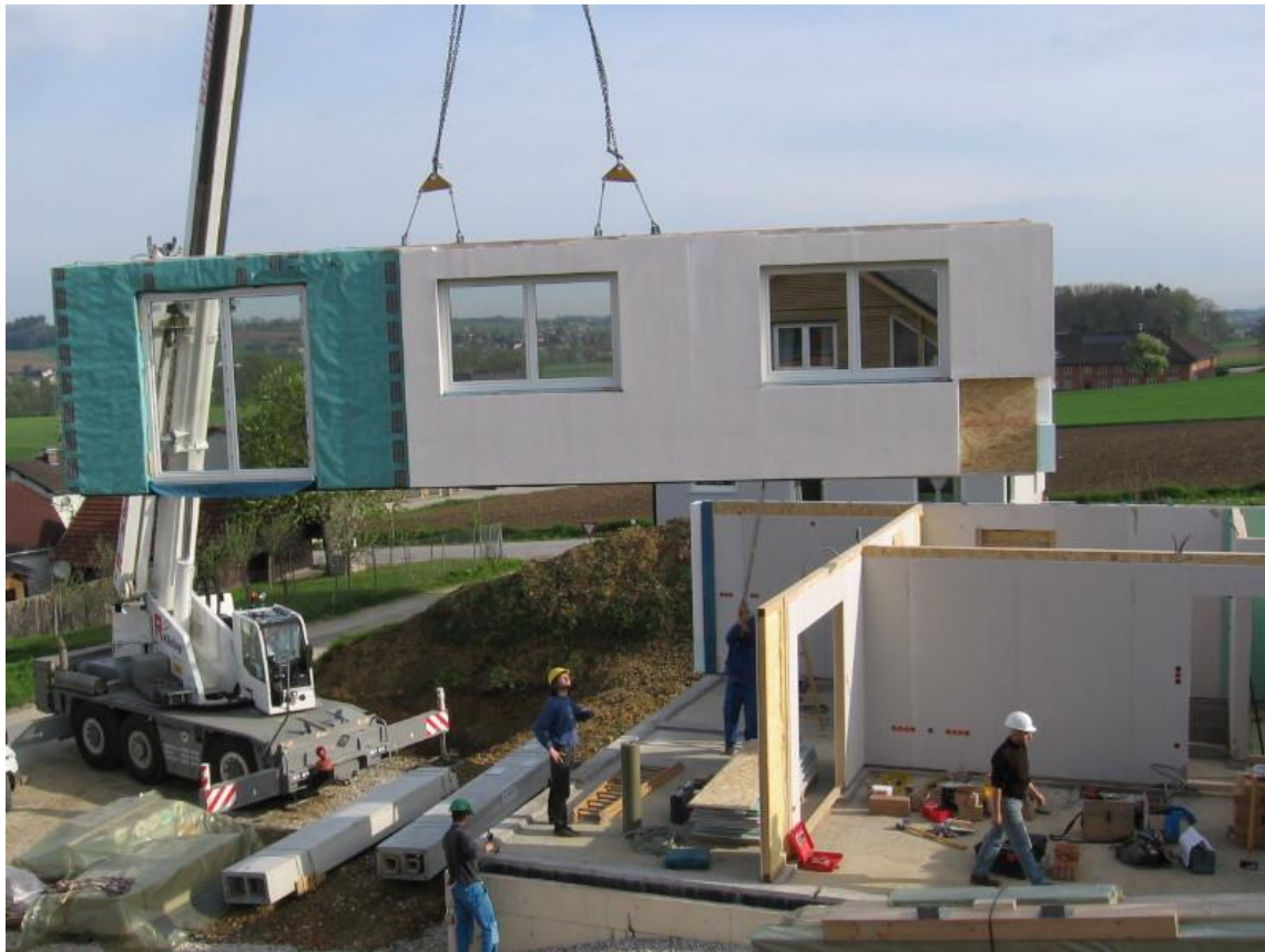
Workers in the UK construct a prefabricated house.
