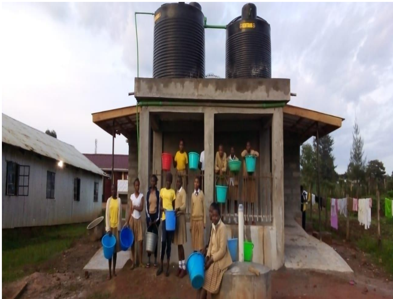
Figure 50: Girls from secondary schools helping themselves with the new WaSH facility provisioned by HOP
