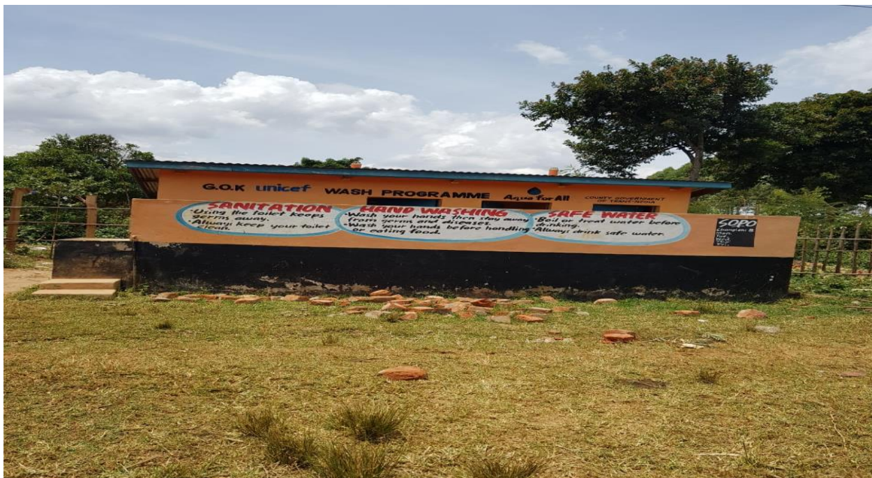
Figure 49: Some examples of government sponsored pit latrines in Mukuyu Primary school
