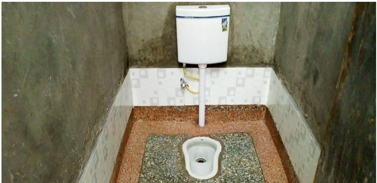
Figure 43: An example of pour flush Sanitation technology provisioned by HOP in Mukuyu primary school
