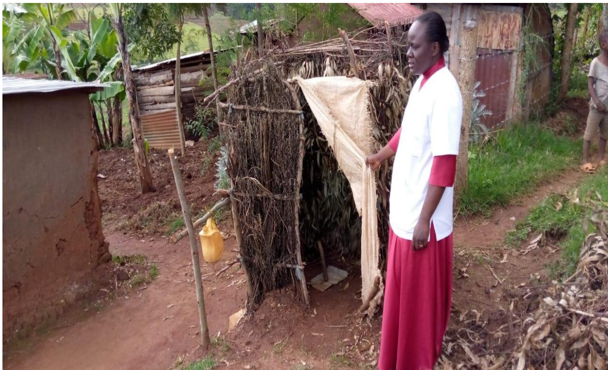
Figure 38: A basic pit latrine made from sticks and old rags (with a hand-washing station made of jerry can)
