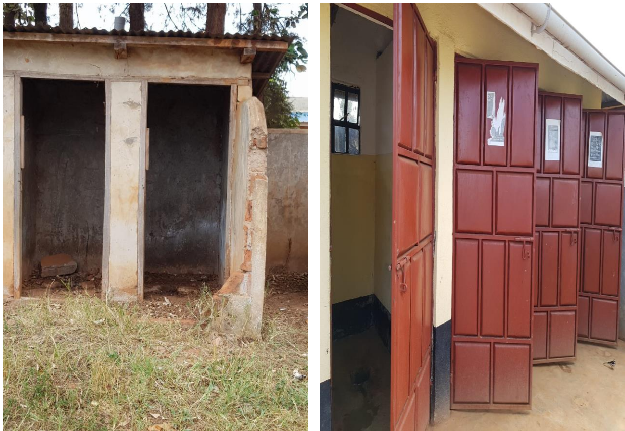
Figure 48: Some examples of government sponsored pit latrines in Mukuyu Primary school
